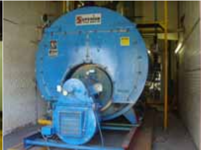
Gas Fired Boiler - 350hp
